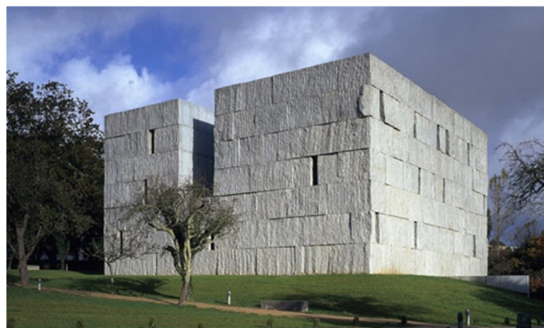
18 Left: Alejandro de la Sota, Civil Government of Tarragona; voids main facade. Right: Antón García-Abril, Centre of Musical Studies; void volume
