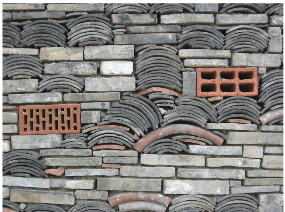
01. Wang Shu and Lu Wenyu, Ningbo Historic Museum, Zhenjiang, China, 2007; Detail of the façade built using the Wa Pan technique.
