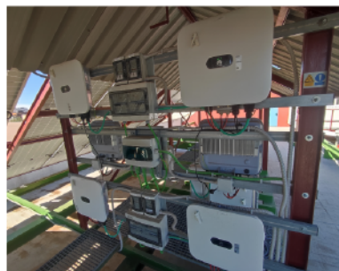
(c) Inversores HUAWEI SUN2000-(6KTL)-M1
