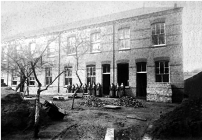
Fig. 03. Sisters outside Brentford Laundry and Preservation Home during construction c. 1894.
